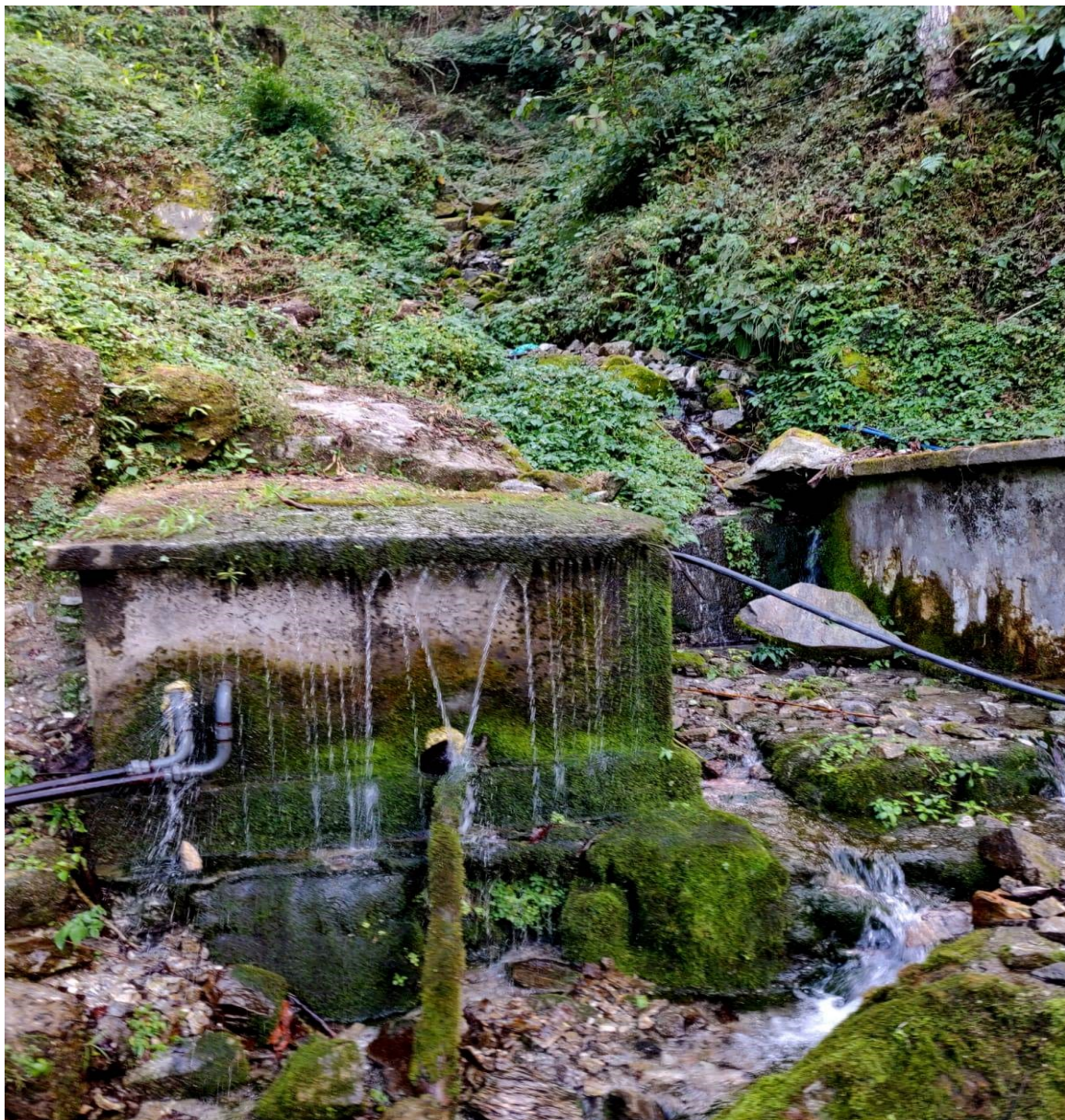
Fig.8.2.2 Spring Box at Darap in Gyalshing block, West Sikkim
